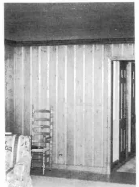
Fig. 5. This photo shows how the entire installation is covered by the vertically sliding panels when it is not in use.
